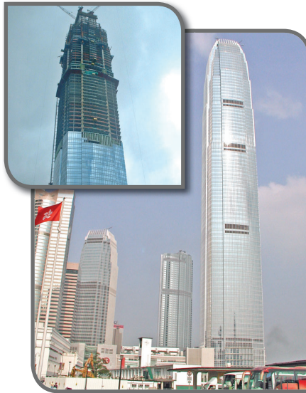
International Finance Centre, Hong Kong
