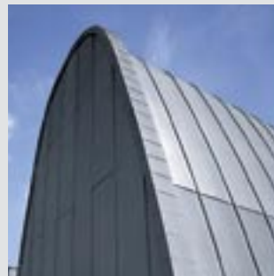
Administration building, Brussels, Belgium
