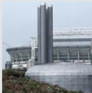
Central heat supply unit, Amsterdam, Netherlands
