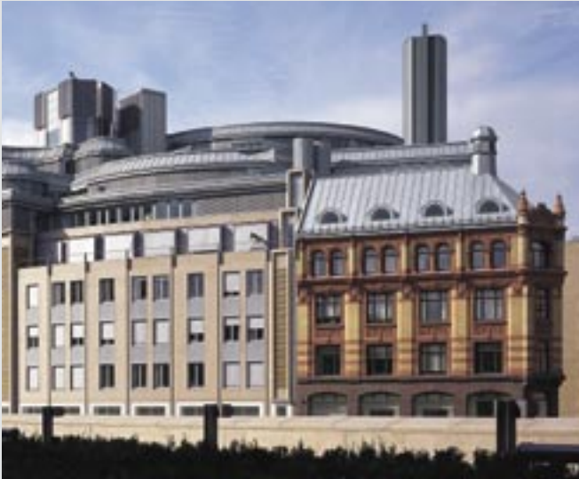
Government building R5, Oslo, Norway
